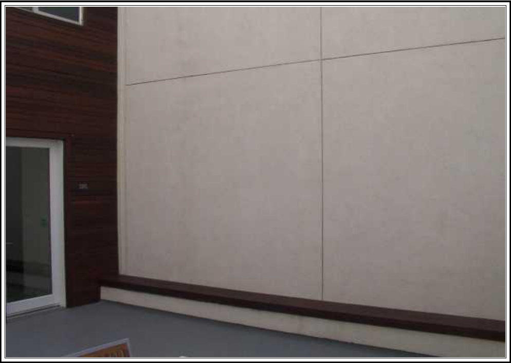
REAR OF SUBJECT PROPERTY
